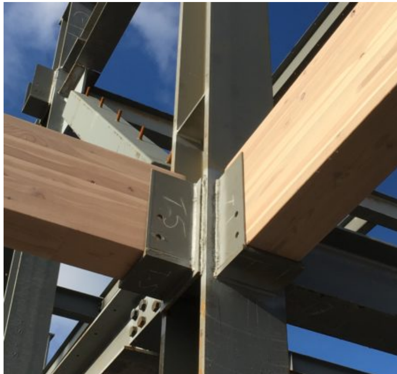
Figure 4: Metal Timber Structures
