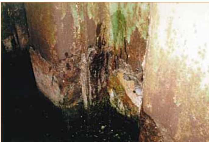
FIGURE 10 - Corrosion de palplanches.
